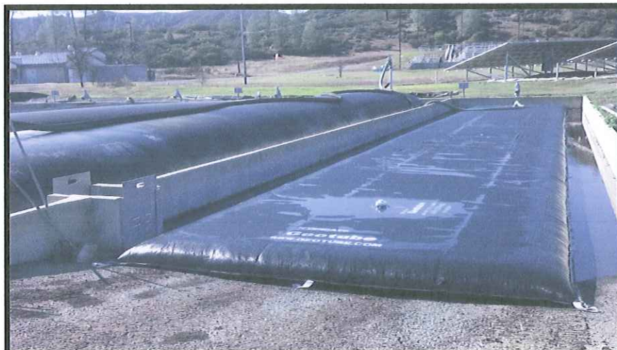
Geo Tube installation in Sludge Bed #6.
