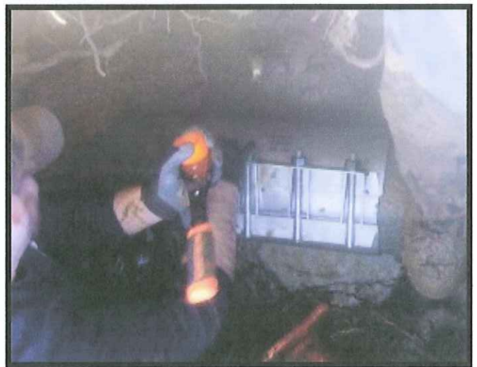
Mainline break repair on Greenridge.
