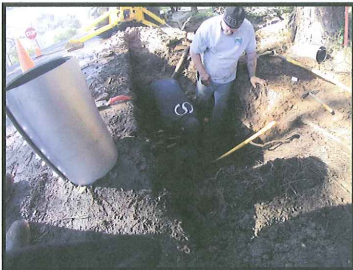
Mainline break repair on Greenridge.
