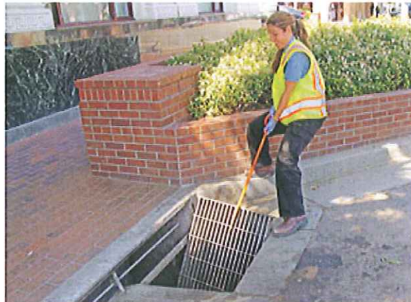
Bill Silverfarb/Daily Journal Debra Bickel, with San Mateo public works, inspects a catch basin filter in downtown San Mateo. The filters keep trash from flowing into local creeks.
