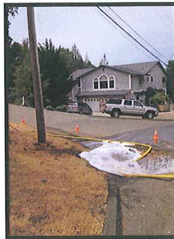
Flushing at Deerhill Road.
