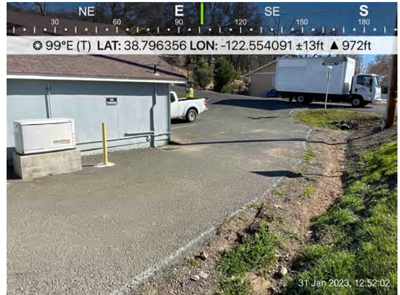
Photo 10. Staging area three, facing east. Photo taken January 31, 2023.
