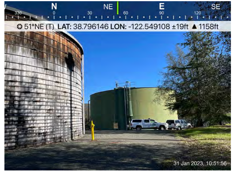
Photo 6. Tank 4 site, facing northeast. Photo taken January 31, 2023.
