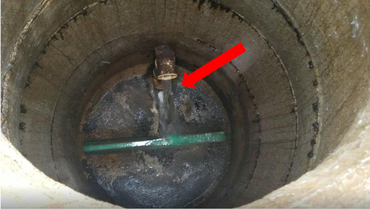
Figure 3: Rain event inspections of manholes (Mountain Meadow South 3.0-6, Hawks Hill 9.5-2).
