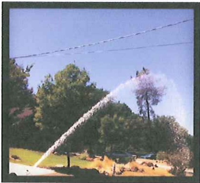
Donkey Hill - Service line leak that was fixed.
