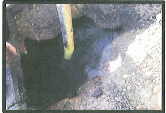
Bear Valley Road - push through for a service connection. The old service connection was leaking.
