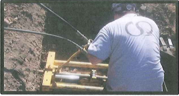
Bear Valley Road - push through for a service connection. The old service connection was leaking.
