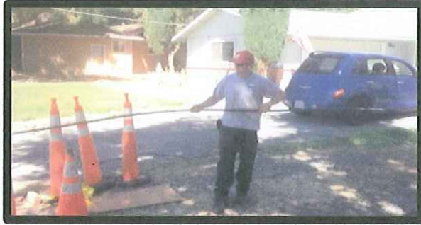
Bear Valley Road - push through for a service connection. The old service connection was leaking.
