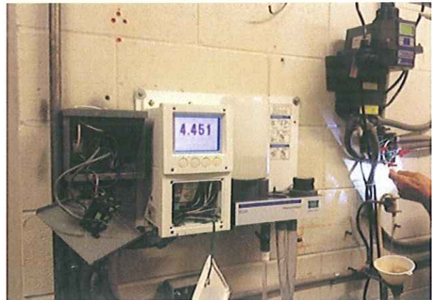
Installation of new chlorine analyzer
