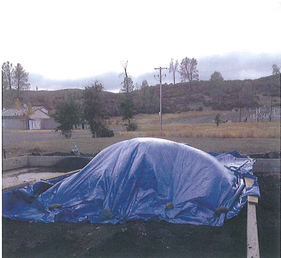
Covered sludge beds in preparation of disposal and keeping the content as dry as possible.
