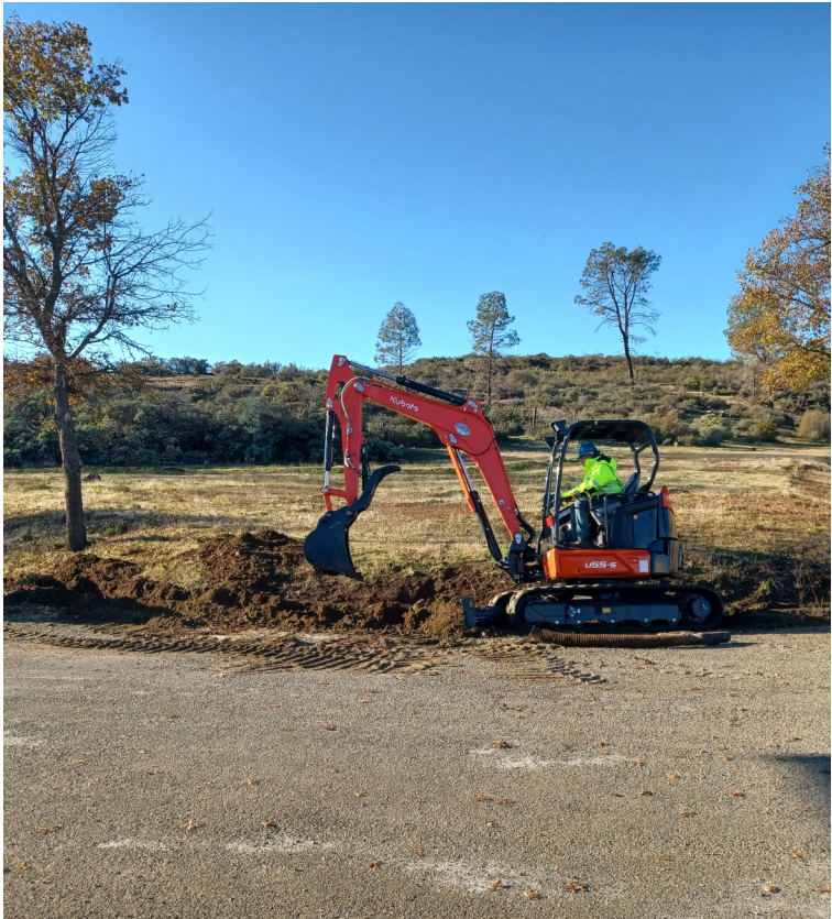
WWTP Drainage Improvements
