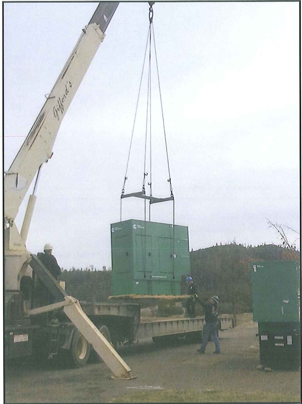
Generator being lifted into place at Lift Station 4.
